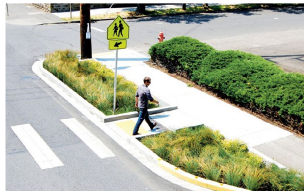
ALL SEGMENTS: STORMWATER PLANTER WITHIN CURB EXTENSIONS
